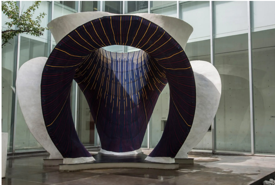
A pavilion constructed using a 3D-knitted formwork developed by Zaha Hadid Architects and ETH Zurich. Photo courtesy of Zaha Hadid Architects and ETH Zurich
