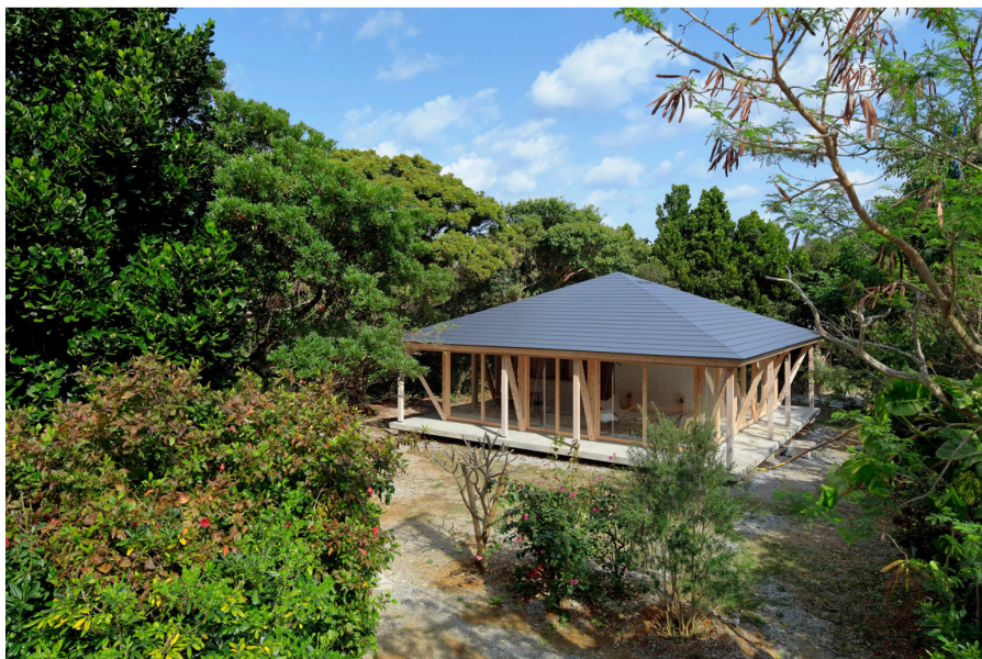
Shinminka House, on Japan's island of Okinawa designed by ISSHO Architects. Designed to withstand devastating typhoon winds while still allowing for cross-ventilation. Photo courtesy of Koichi Torimura
